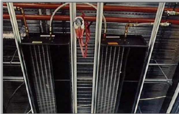
Figure 4 – Recessed Passive Chilled Beams
