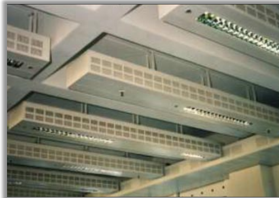
Figure 3 – Exposed Passive Chilled Beams
